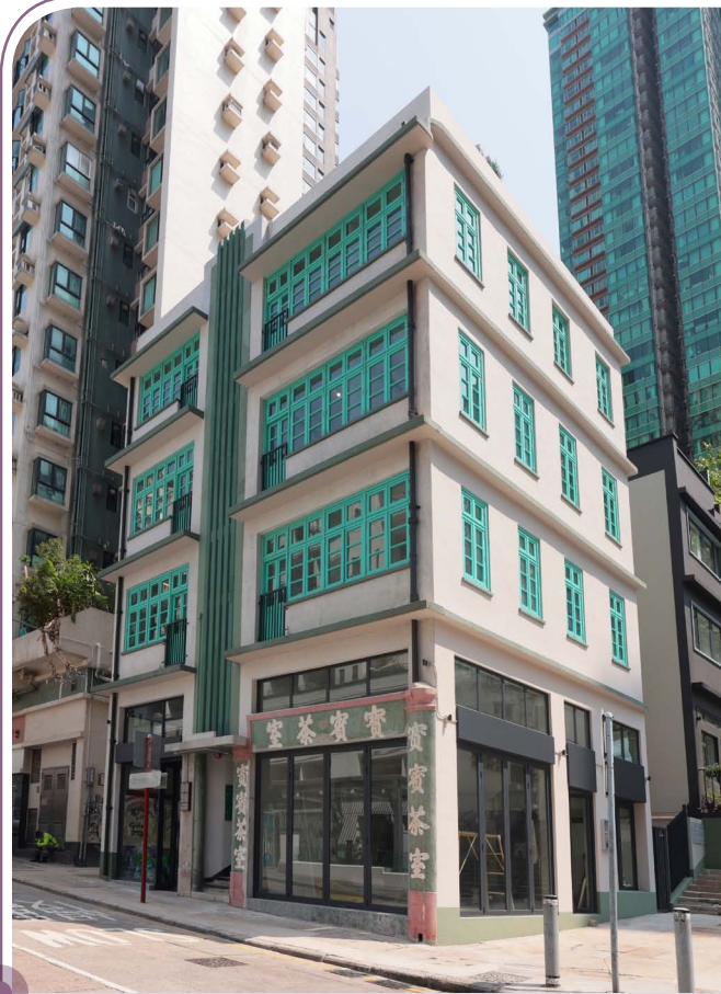
88-90 Staunton Street (Grade II historic building) after rehabilitation, with key features such as Shanghai plaster facades and a terrazzo plaque “寶實茶室” preserved and restored
