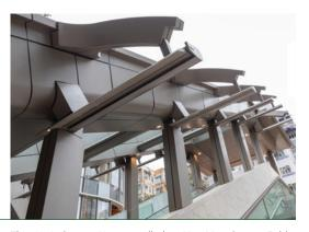
The Air Induction Units installed at Yue Man Square Public Transport Interchange help improve airflow while consuming less energy.
